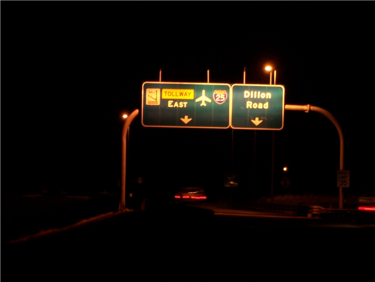
This is an example of a road sign, properly lit, setup by the state of Colorado. The lights are shielded and illuminate the sign with no stray light.
