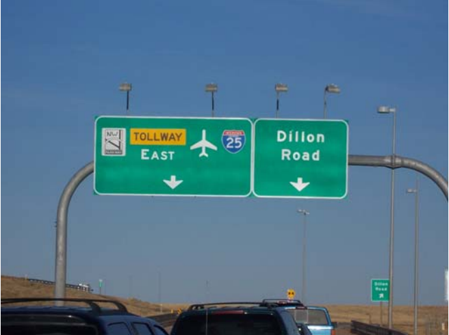
This is an example of a road sign, properly lit, setup by the state of Colorado. The lights are shielded and illuminate the sign with no stray light.
